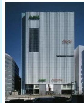
Shinjuku 3-Chome East Building
