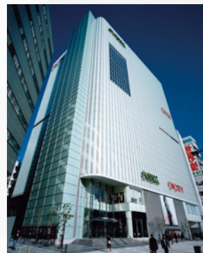
Shinjuku 3-Chome East Building
